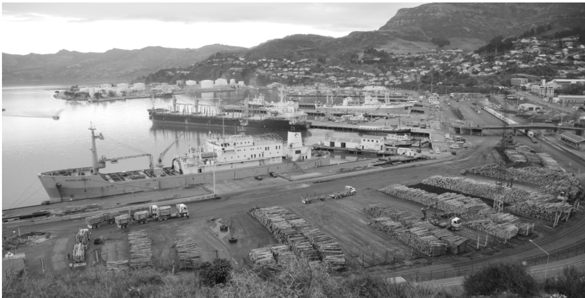
The NZCPS makes special provisions for ports and port operations such as the Port of Lyttelton (pictured here) in recognition of their contribution to transport networks and the economy.
